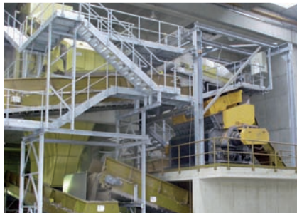
Application: Packaging, rejects, matured timber, screen overflow Solution: XR3000 Location: Austria
