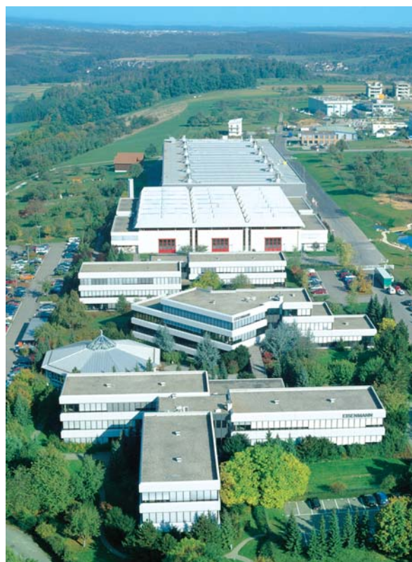
EISENMANN technology center in Holzgerlingen
