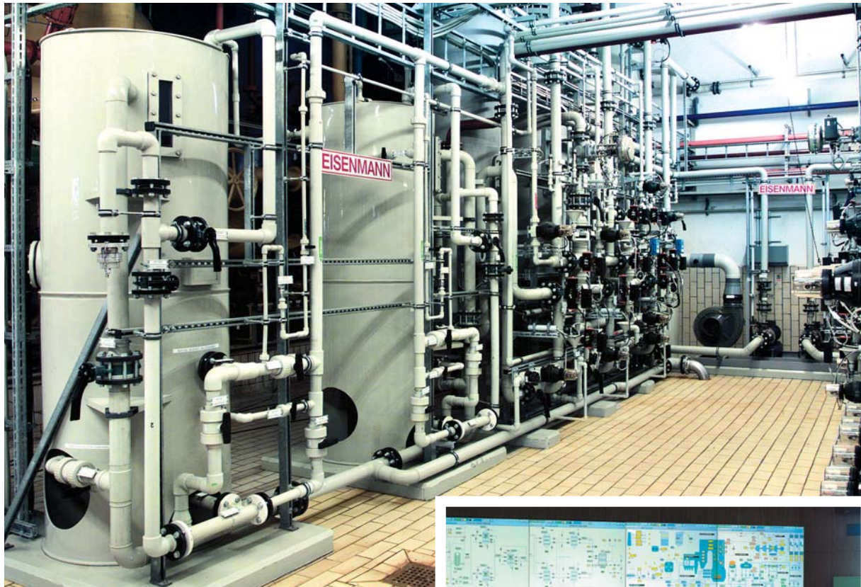
Top: Ion exchanger fluidized bed system for water purification in a power station
