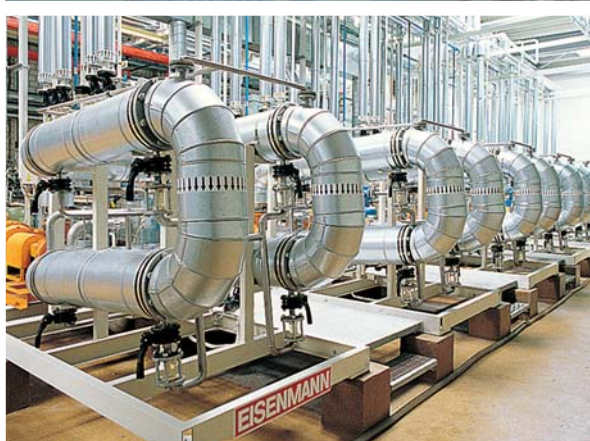
Top: Ultrafiltration system for emulsion splitting at a liquid waste disposal company.
