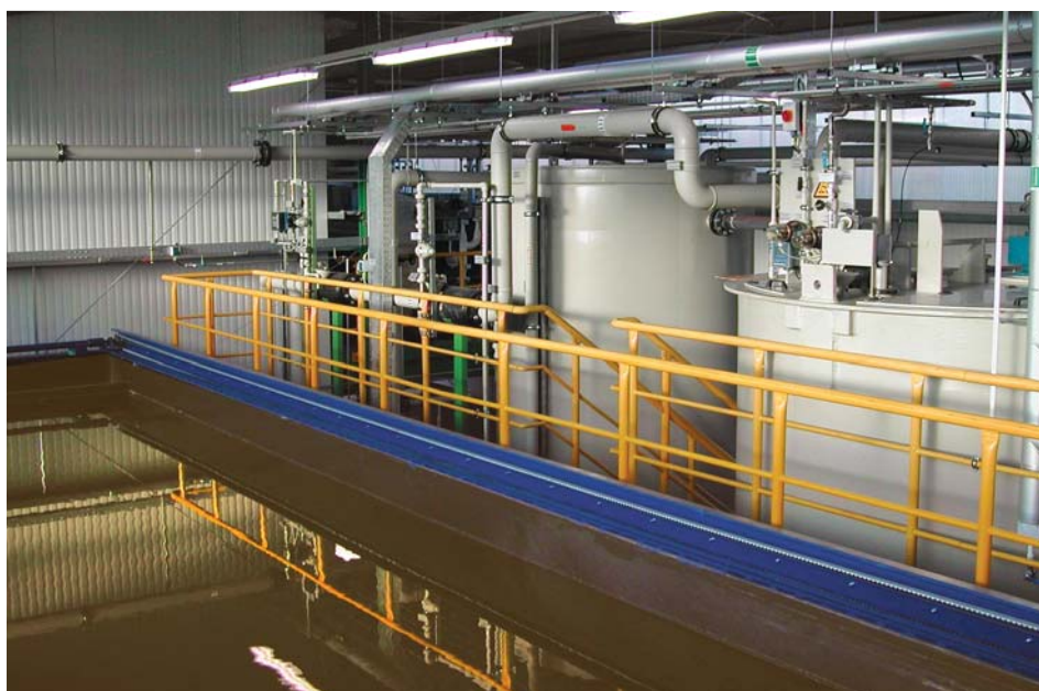
Waste water treatment for direct discharge in a river: Phosphate precipitation with contact sludge recirculation and a high-performance sludge clarifier for a chemical production plant
