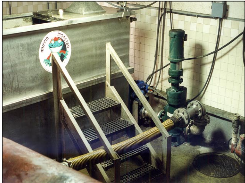
Clogs and jams are eliminated thanks to the integration of the powerful and very hungry Muffin Monster grinder.
