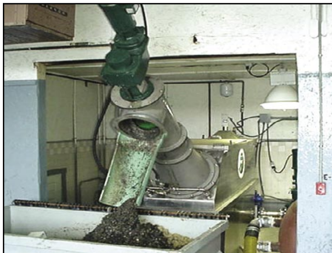
The Honey Monster grinds, washes and screens solids, reducing odor and decreasing volume.
