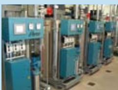
the MULTIPLE STEAM GENERATING UNIT MDA
