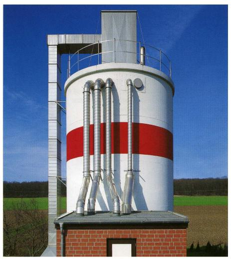
Silo-top-filters series B05, B07 for installation in filter rooms and outside in accordance with the safety rules and the TRGS 553 of the HBG (German standards) for the extraction and separation of wood dust and wood chips. Further information is available in the leaflet ZH 1/728 "Silos for wood dust and chips" of the Holzberufsgenossenschaft (Employers' Liability Insurance).
