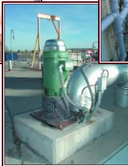
Primary Clarifier Scum
