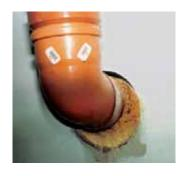
The annular gap around a pipe is sealed with foam. Foam loses its dimensional stability over the course of time and the seal is therefore not tight.
