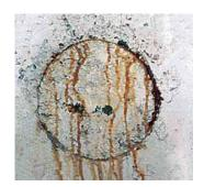
A core bore that is no longer required cannot simply be refilled using the existing core; this closure is not watertight.
