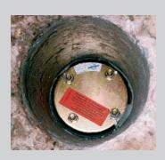
An optimum solution here is a blind Curaflex® C gasket insert with Aquagard sealant applied to the inside of the core bore.
