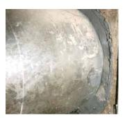
When the pipe moves due to temperature fluctuations, in the case of mortar-embedded pipes pictured here, cracks between the pipe and surrounding concrete occur, and the duct loses its seal.
