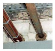
Fire regulations should have been taken into account when both these pipes were passed through the wall. The arrangement in the left-hand picture would allow smoke, fumes and flames to penetrate the opening.
