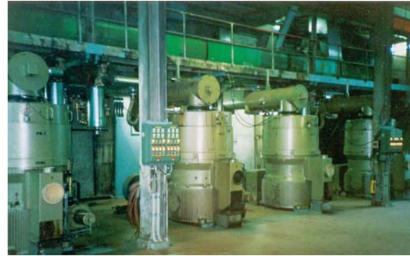
Pelleting plant with 4 presses
