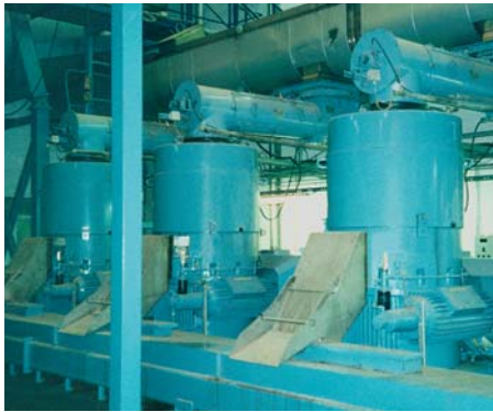
Pelleting presses in a sugar factory
